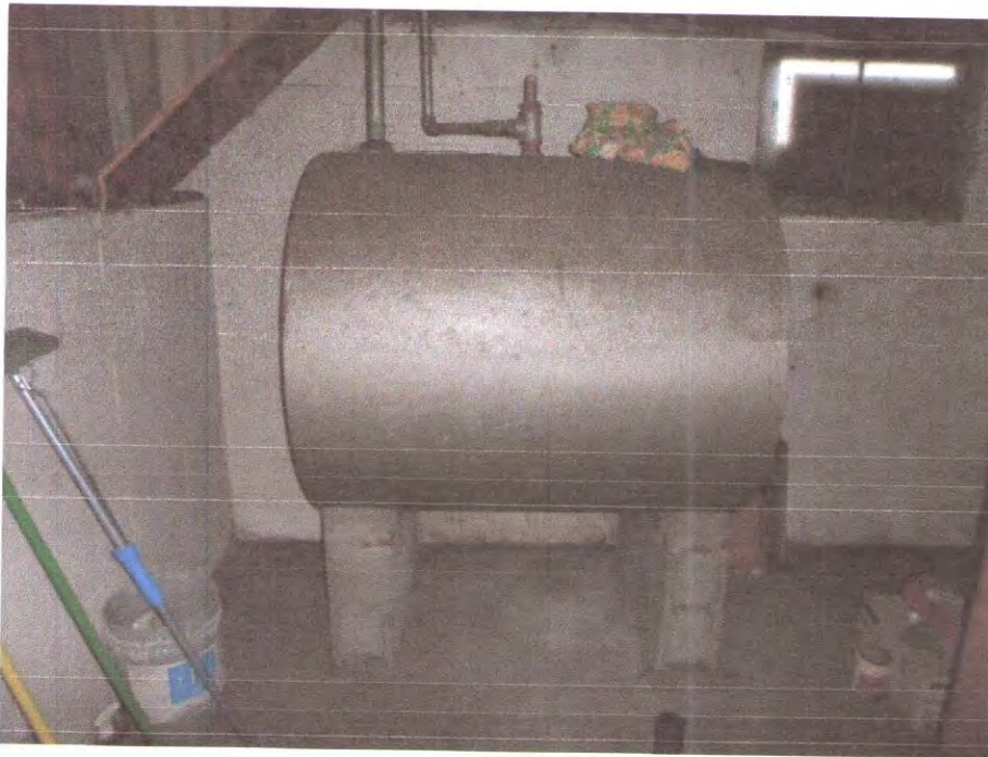
1. Photograph depicting the fuel oil AST located in the basement of the residence.
